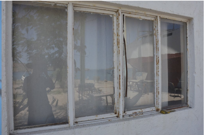
Condition of Windows
