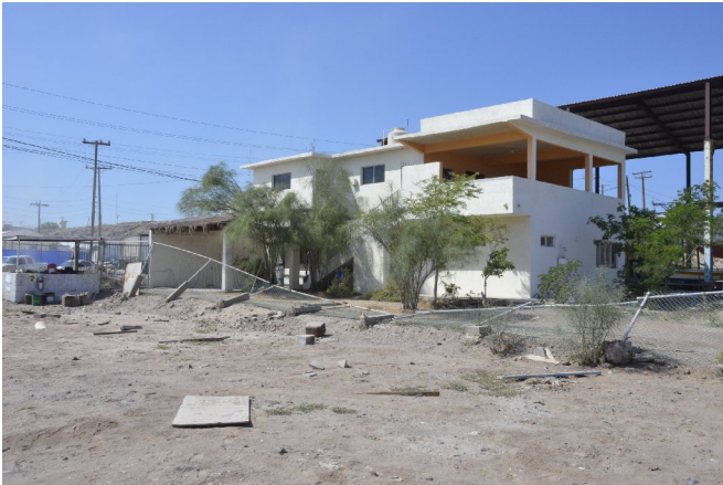
View of the house
