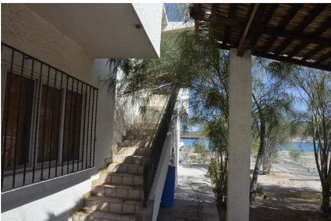
Stairs blocked by thornbush
